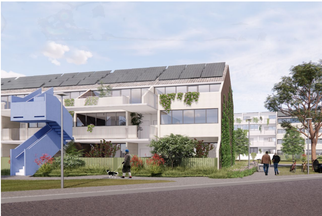
View of the refurbishment of Barack Beacon with photovoltaic cells retrofitted to the north oriented rooftops. Image by OFFICE
