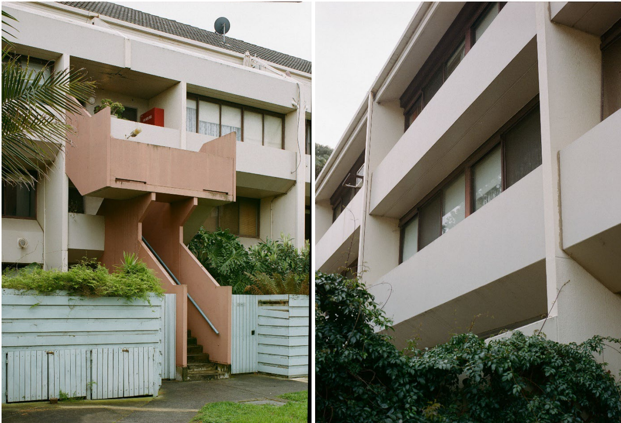
The existing homes at Barak Beacon, constructed from precast concrete, were built in 1982 by the Ministry of Housing. Photos by Ben Hosking
