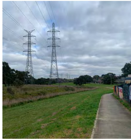
Powerline Easement Intersecting Waterway
