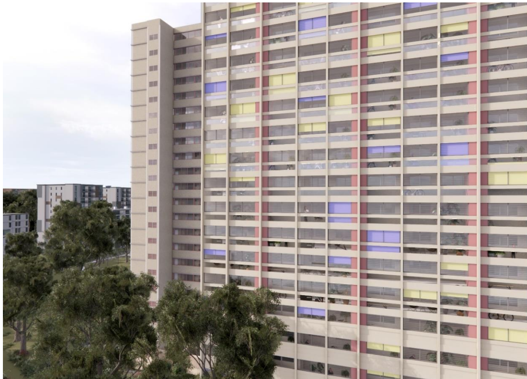
View of the west facing facade with new prefabricated concrete balconies, louvre windows and colour retractable blinds. Image by OFFICE
