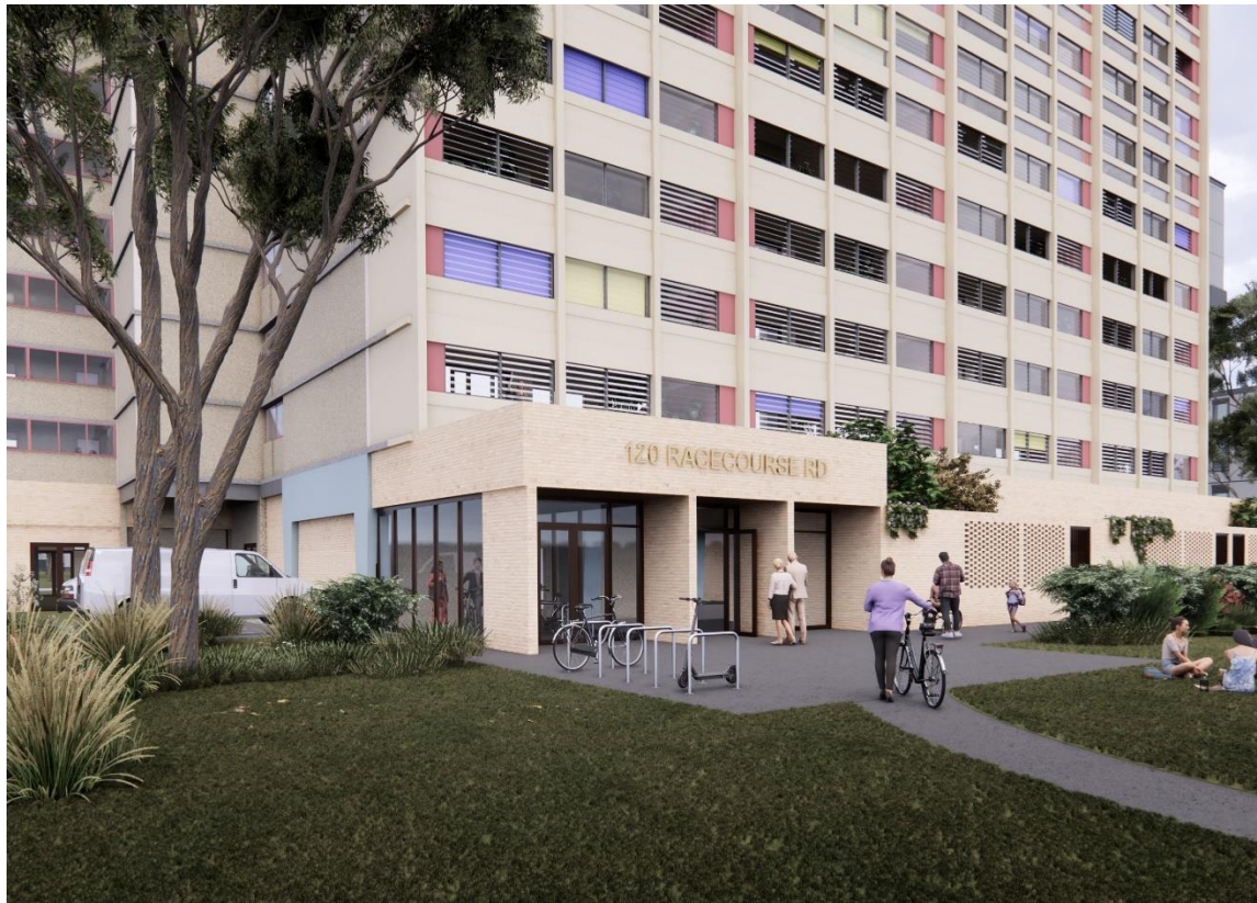
View of the RRR proposal shows a new cream brick entry and SDA units on the ground floor. Above are the new prefabricated concrete balconies with glass louvers for passive heat and cooling, as well as safety. Image by OFFICE.
