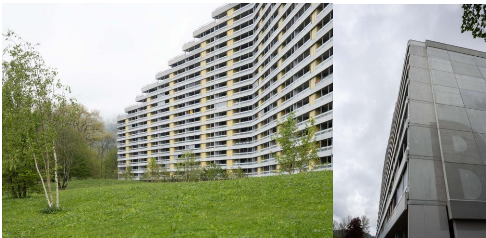
The prefabricated concrete balconies integrate into the existing building fabric while giving the façade a refresh. Photo by OFFICE.
