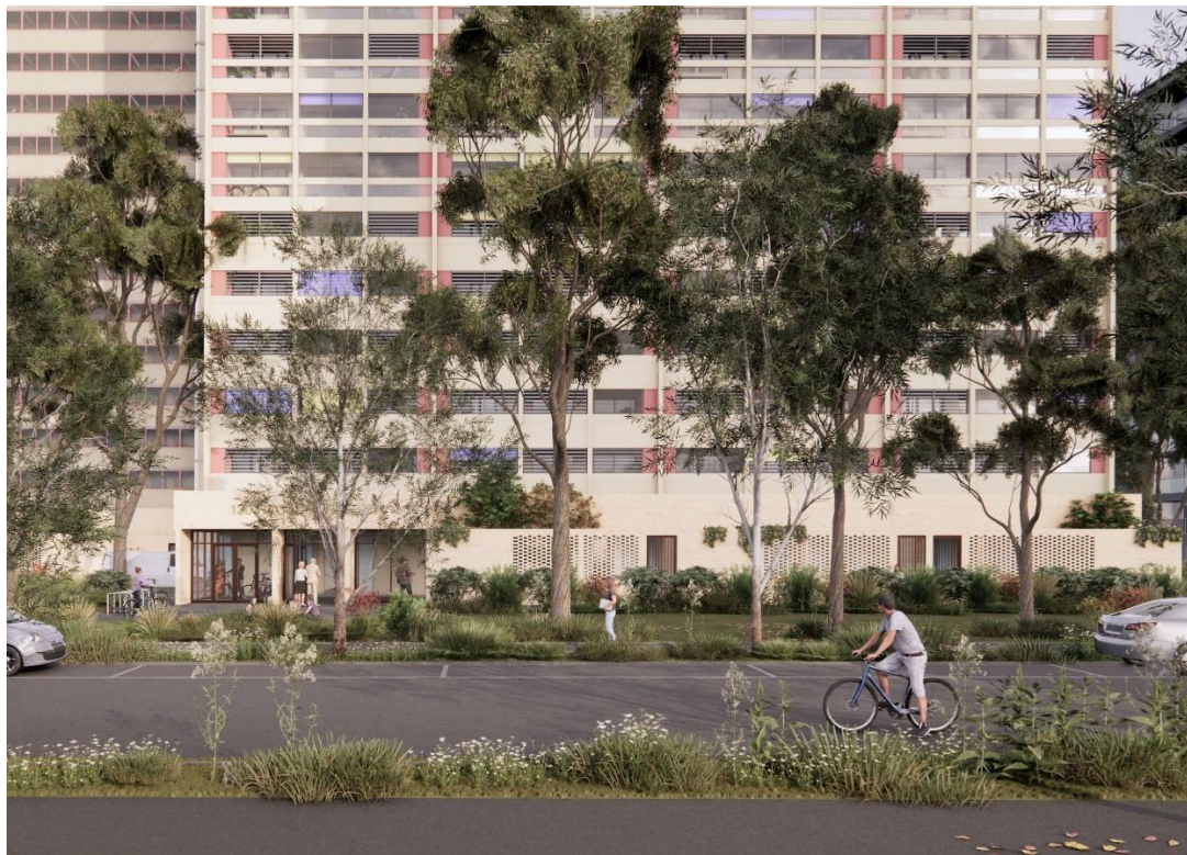
Render of the retrofitted Flemington Towers with brick base and new balconies. Image by OFFICE.
