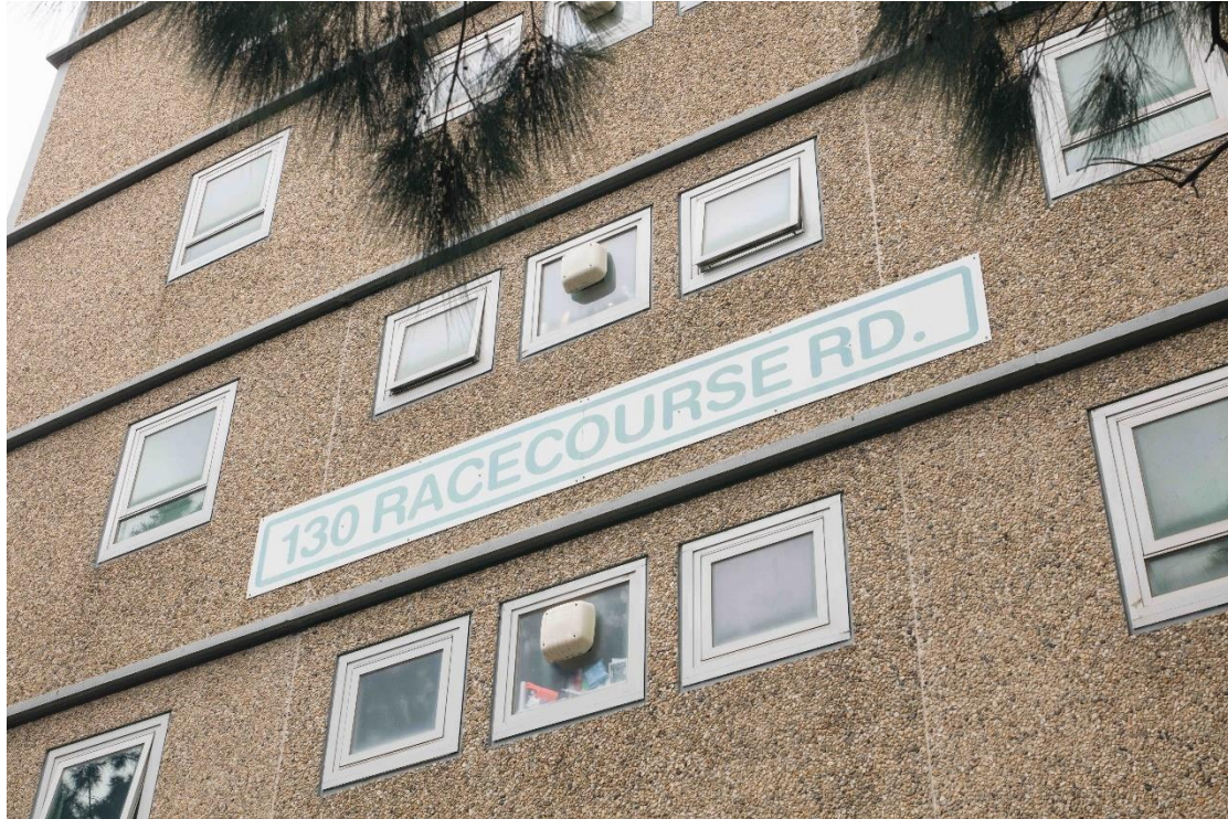
130 Racecourse Road will be demolished as part of the High-Rise Redevelopment Program. Photo by Ben Hosking.
