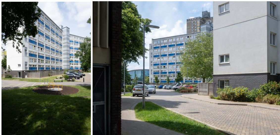
Over cladding to the existing estate building have drastically increased the thermal performance, allowed for structural maintenance and reinvested the identity of the building for the residents. Photos by OFFICE.
