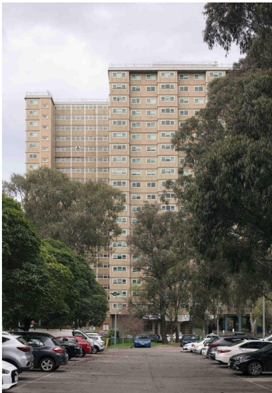
The thoughtful design and layout of flats allows for every room to have a window and cross ventilation. Visually, the towers show no signs of cracking or spalling. Photo by Ben Hosking.
