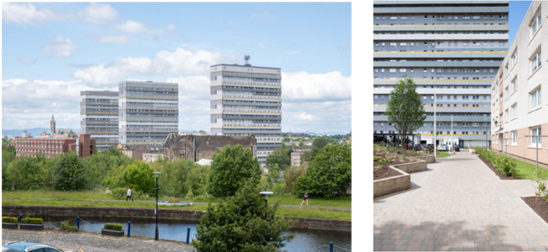
Photo of the refurbished towers at Cedar Court Estate in Glasgow. Photo by OFFICE.
