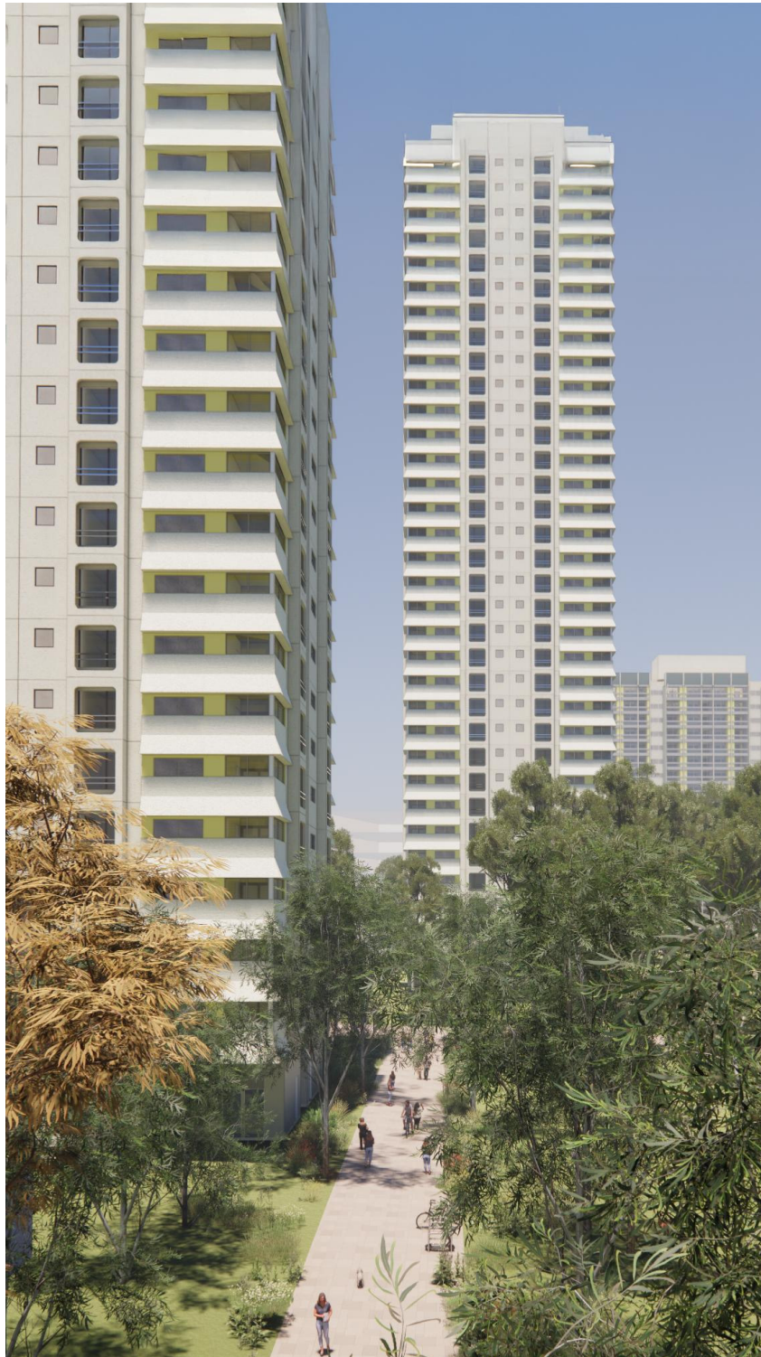
Render view towards Matavai and Turanga showing retrofitted balconies with sun shading and louvres. Image by OFFICE.
