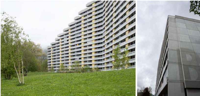
The prefabricated concrete balconies integrate into the existing building fabric while giving the façade a refresh. Photo by OFFICE.
